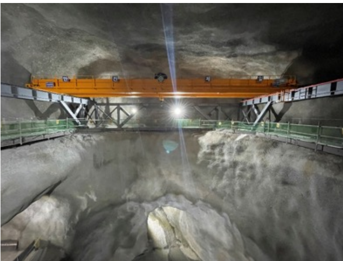
LSC Hall 10-ton crane • Completion June 2023
